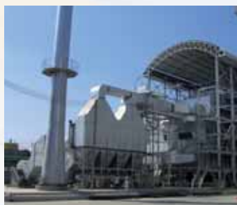
Bua Yai Bio Power Plant, Thailand Biomass/Agriculture Industry
